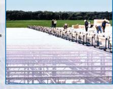
however, eliminate the fall hazard from the perimeter of the roof. OSHA document 29 CFR 1926 (u) (3), requires that workers be protected from falls along all roof edges to which they are exposed. Quality assurance testing, witnessed by an independent consulting firm, provided verification of the system's capabilities.
